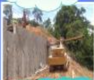
Soil Nail Drilling Machine
